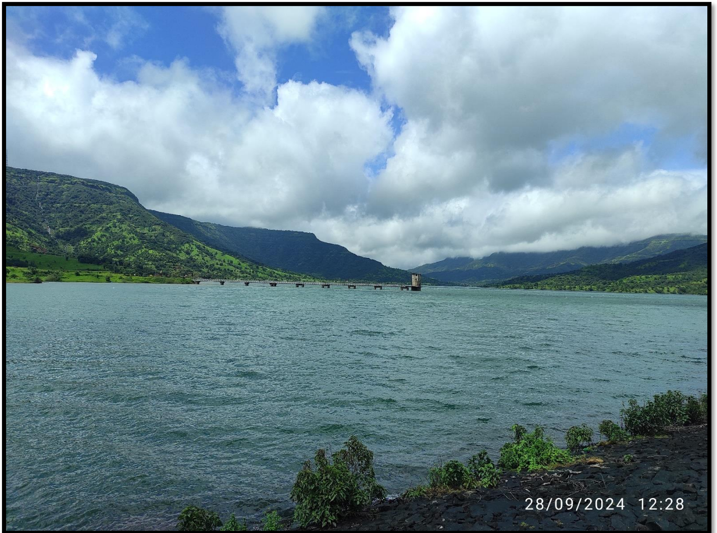
Fig. 9: View of backwater stored in reservoir in upstream side (Mahabaleshwar side)
