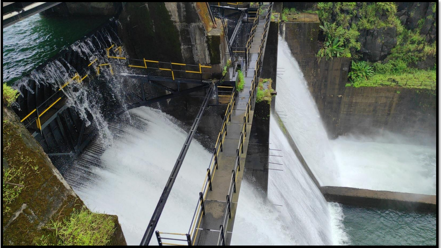
Fig. 6: Discharge from 3 radial gates of Dam. Gates are operated with electric power and can be operated manually too. They demonstrated its control and operation thoroughly.
