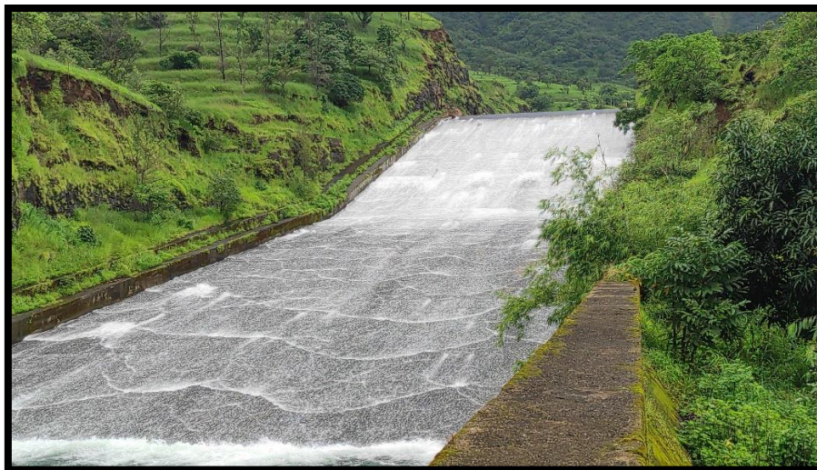
Fig. 28,29: Water released from Spillway of dam (photo 6, 7) comes down further with high velocity due to slope and we need to dissipate its energy to avoid erosion further so such type of design is made so that hydraulic jump will be formed and excess energy will be released before water meets river course at normal elevation. Its very much interesting to know all these technical points minutely and from application point of view. The energy dissipation structures like Stilling Basins, Flip Buckets, Plunge Pools, Baffle Blocks are crucial for reducing the kinetic energy of water released from the dam to prevent erosion, structural damage, and downstream flooding.
