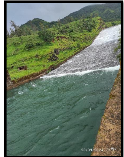
Fig. 28,29: Water released from Spillway of dam (photo 6, 7) comes down further with high velocity due to slope and we need to dissipate its energy to avoid erosion further so such type of design is made so that hydraulic jump will be formed and excess energy will be released before water meets river course at normal elevation. Its very much interesting to know all these technical points minutely and from application point of view. The energy dissipation structures like Stilling Basins, Flip Buckets, Plunge Pools, Baffle Blocks are crucial for reducing the kinetic energy of water released from the dam to prevent erosion, structural damage, and downstream flooding.
