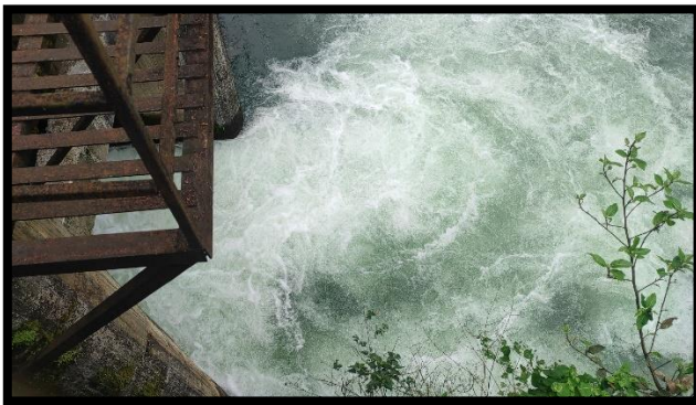
Fig. 24,25: Water coming out of Power plant from depth through Draft tube and going further to downstream side in River.
